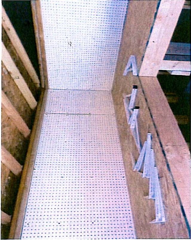
Upper Shelf Installation and Lower Shelf Liner
